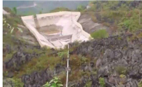
Fig 2. A concrete tank without water during the dry seasons in DVKP
